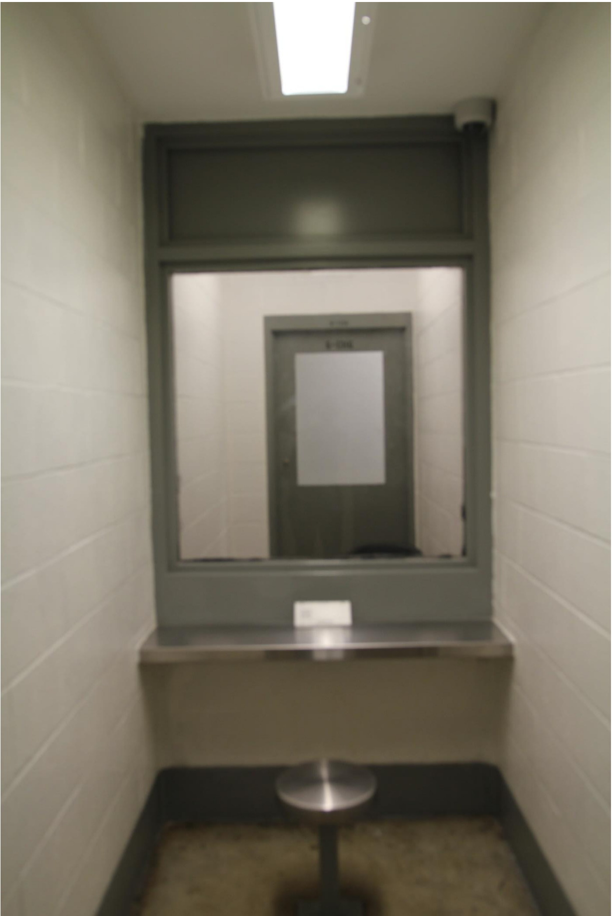
Image 26: Standard no-contact SMU visitation booth. A sealed Lexan panel separates the visitor from the prisoner. Conversation takes place through an electronic box mounted just below the window.
